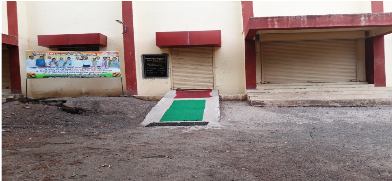
Ramp for Differently Abled Students
