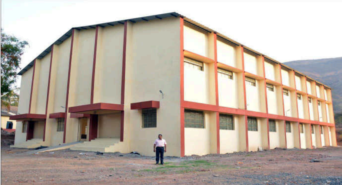
Indoor Sport Hall (External View)
