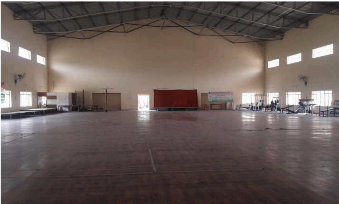
Indoor Sport Hall (Internal View)
